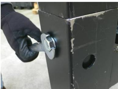
Tighten the two screws with a good torque in order to ensure a steady connection.
