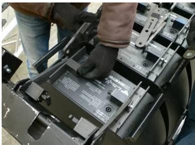
Connect the frame to the first loudspeaker by means of the two bars previously connected (point 9).
