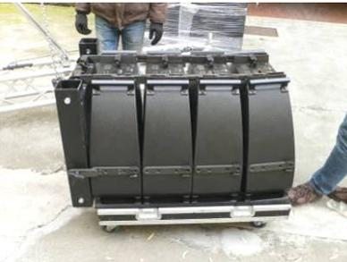
When the last module is on the dolly, **before proceeding with the following steps, please be sure that the chain connected to the motor is NOT under tension. Otherwise you must lower the motor, so that no load is taken by the lifting point.**
