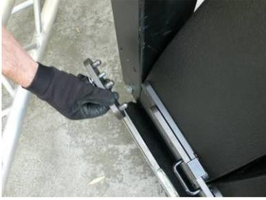
Insert the side connecting bar into its location.
