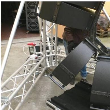
Lift the system and connect the side bars on the loudspeakers following the same procedure shown for the previous group. Repeat the operations from #22 to #31 in order to complete the installation of the line array.
