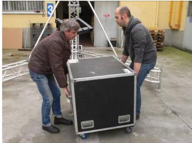
Move the flight-case with the loudspeaker close to the rigging structure.
