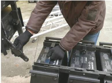
Remove the back bar from the first loudspeaker on the dolly from the flown system. Repeat steps 34, 35 and 36 for the remaining blocks of loudspeakers.
